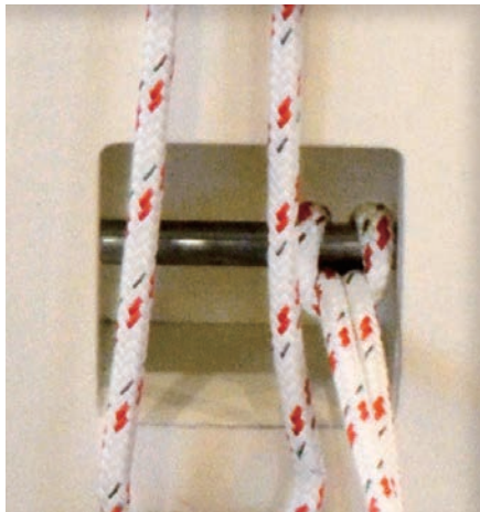
4. Attachment: A box built into the wall with a steel bar secured in the middle.
